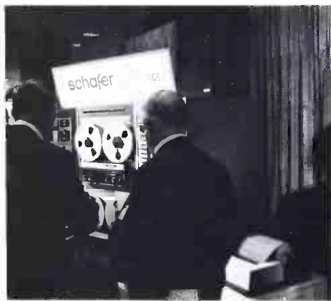
Automation equipment was big.
